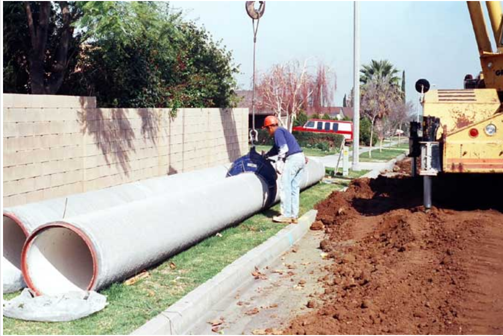
Safe and easy to attach, Stemar pipe tongs release automatically when the pipe is in position.
