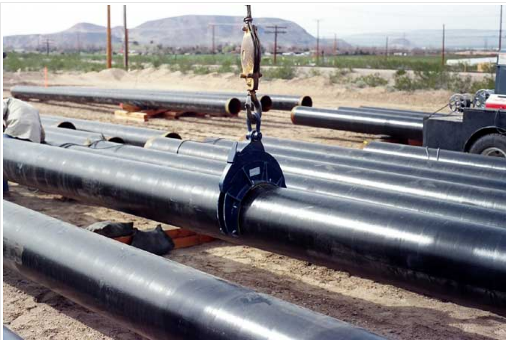
16" Steel pipe tong with special belting liners to protect pipe coating.
